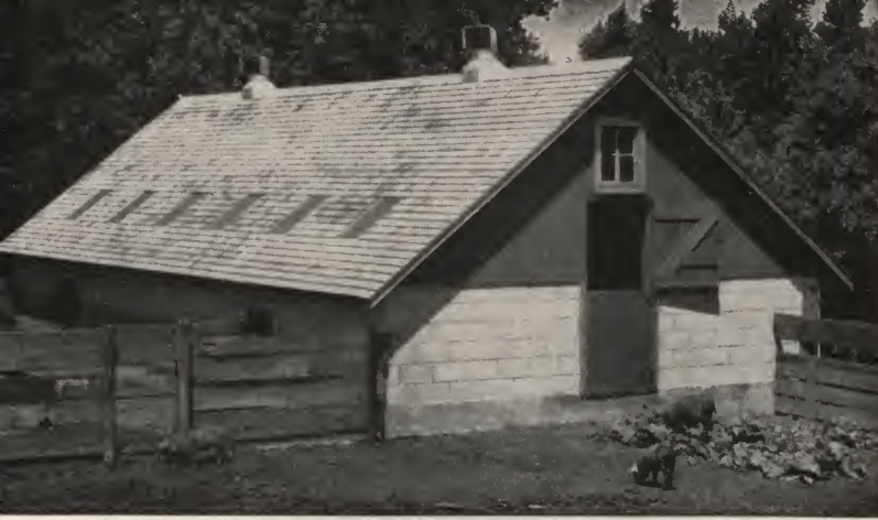
Good examples of the modern gable roof and gambrel roof hog houses. Houses like these in the northern half of the United States should have insulated ceilings about 7 ft. 6 in. above the floor to provide a warm house for early spring farrowings.
